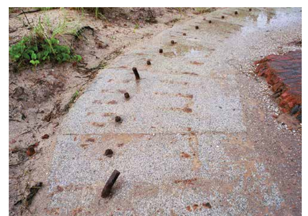
Bolts that held the iron Lighthouse to the granite foundation can be seen
