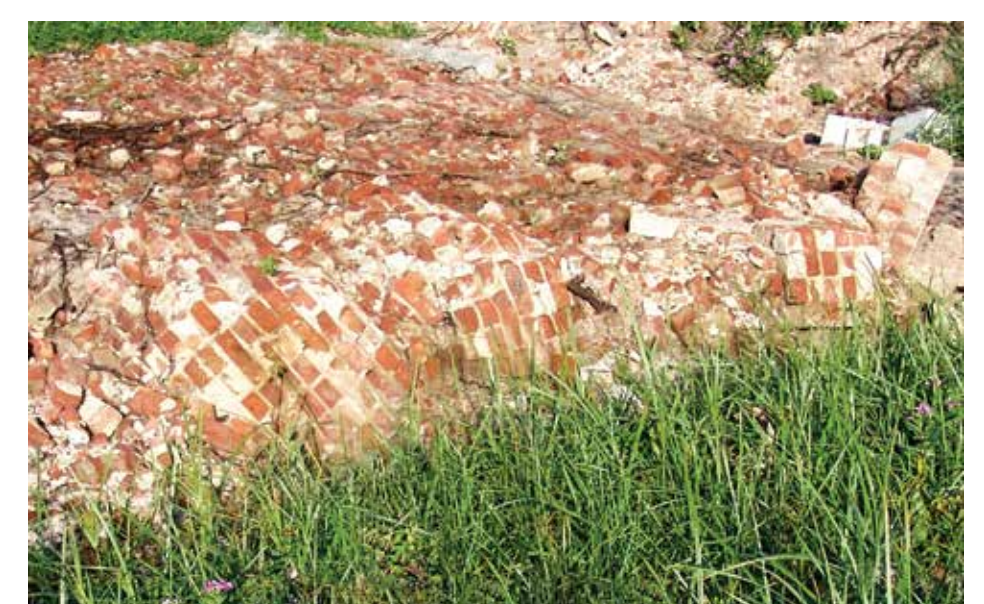
Site of the first Lighthouse, blown up to make foundation for new site of the iron lighthouse
