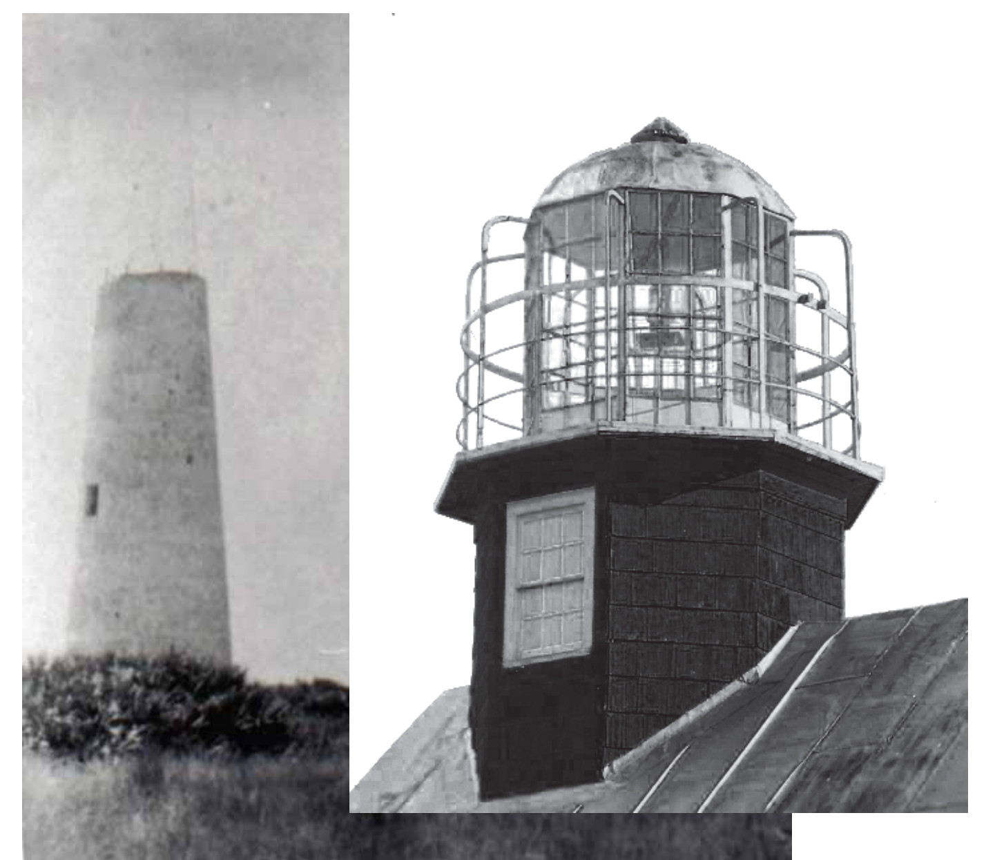
1848 brick tower and example of a birdcage-style lamproom similar to the one originally on the top.
