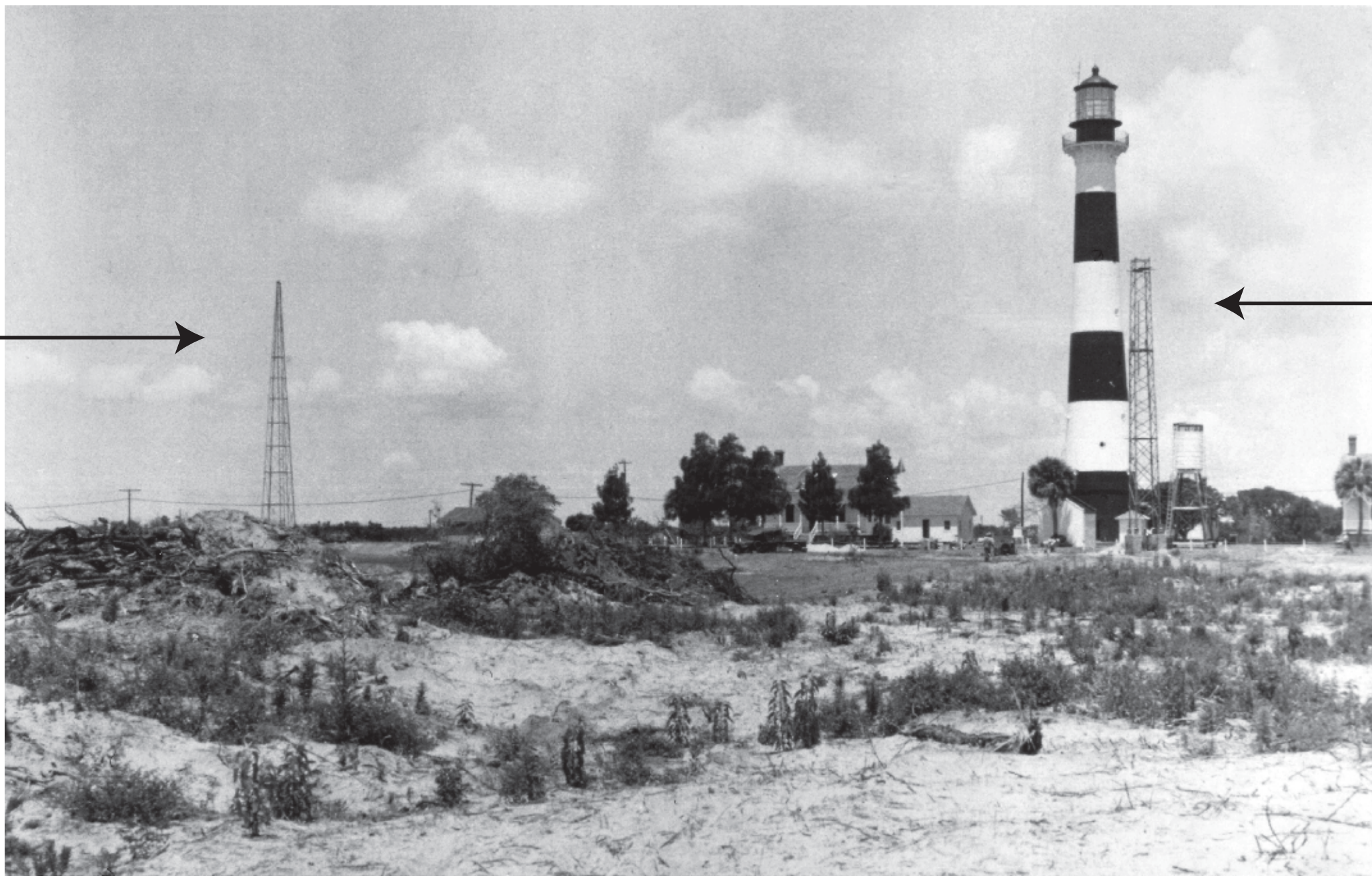
The original 1931 radio tower can be seen at far left. A new 1950 radio tower is under construction just to the right of Lighthouse.
