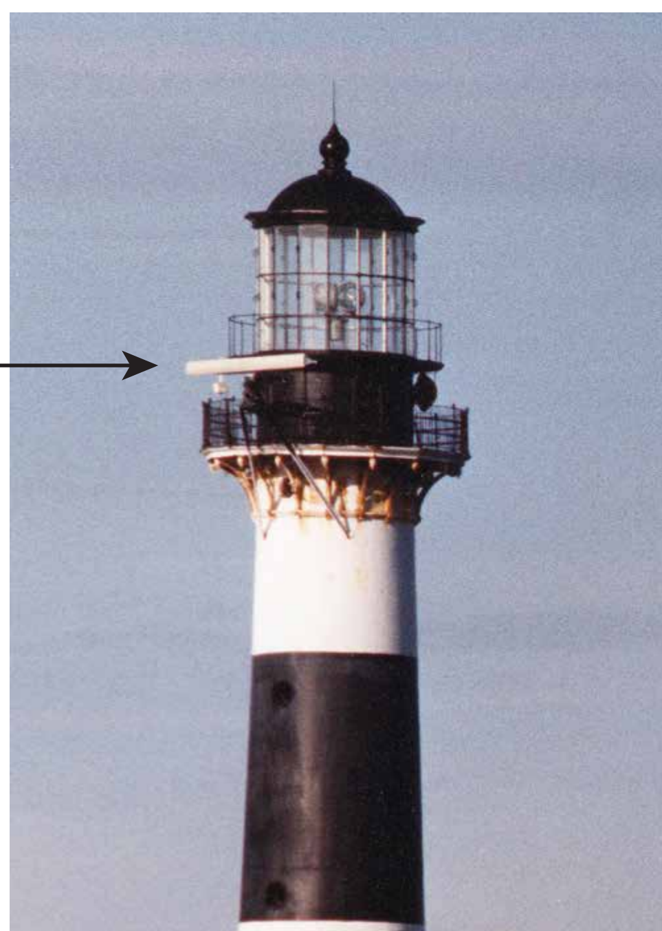
Attached to the lamp room on the left is the horizontal 1969 radar antenna.
