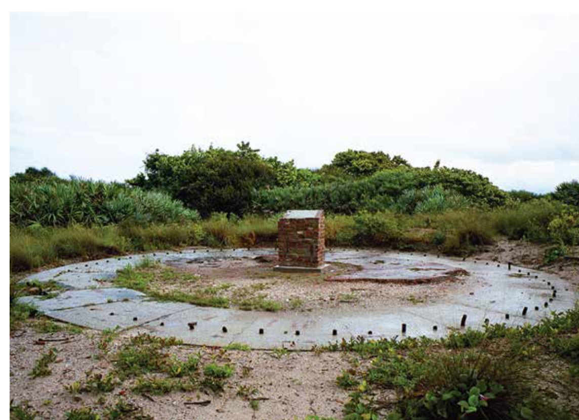
Original granite foundation on first site of the iron Lighthouse
