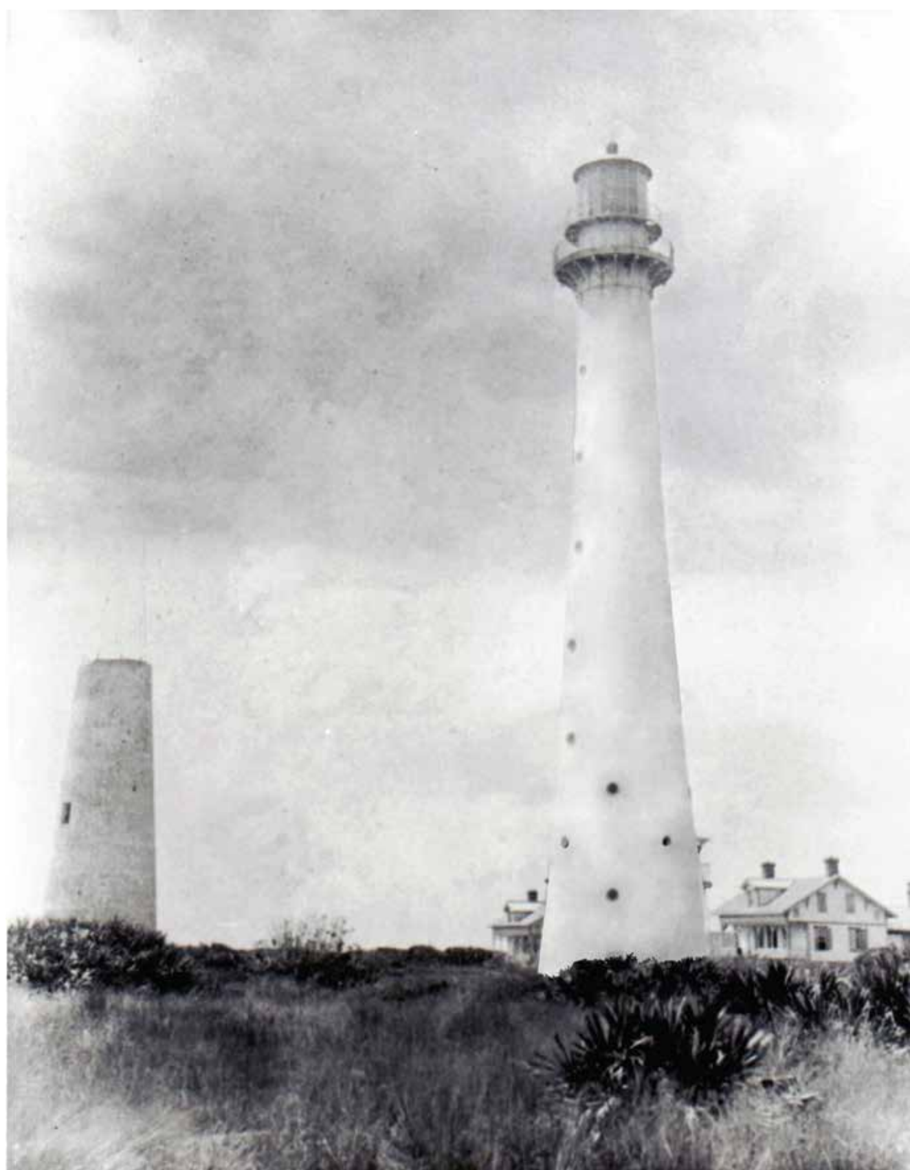
The new iron Lighthouse looks down on the old tower
