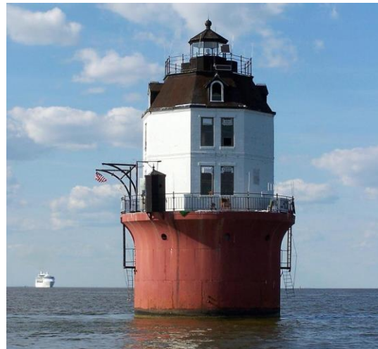
Caisson Baltimore Harbor Light, Maryland (the lighthouse sits on a large concrete block sunk into the seabed)
